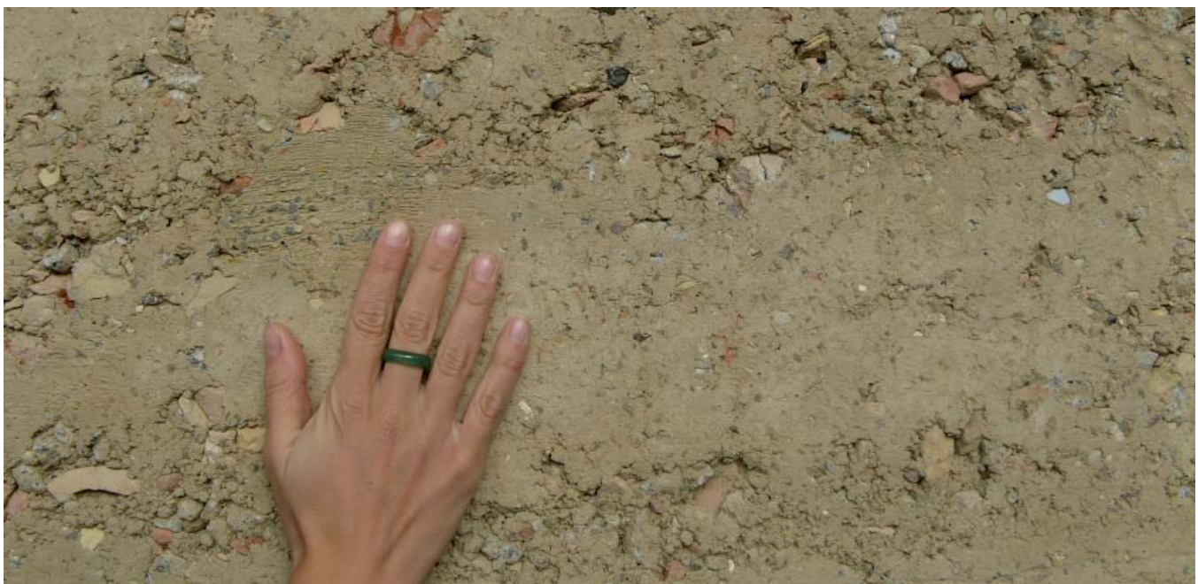
Rammed Earth Construction
